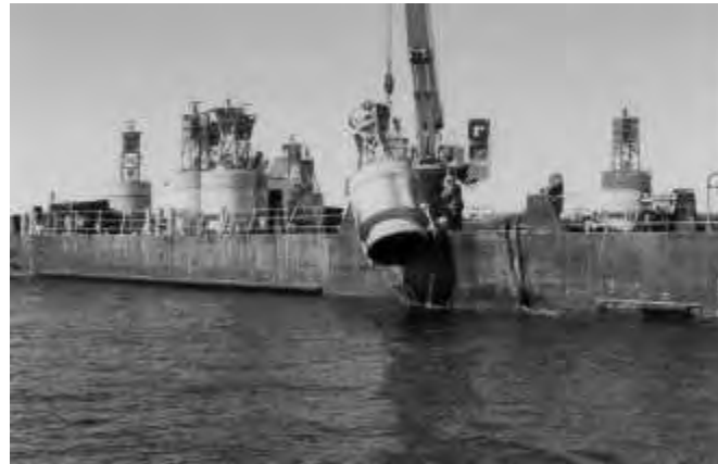
SLSDC maintenance staff place navigation aids along the St. Lawrence River using DGPS technologies.
